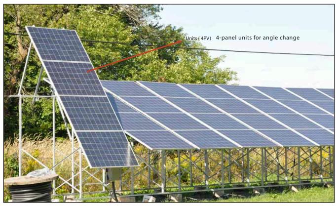
Ground Mount aluminium, adjustable and adaptable to different types of PV solar.
